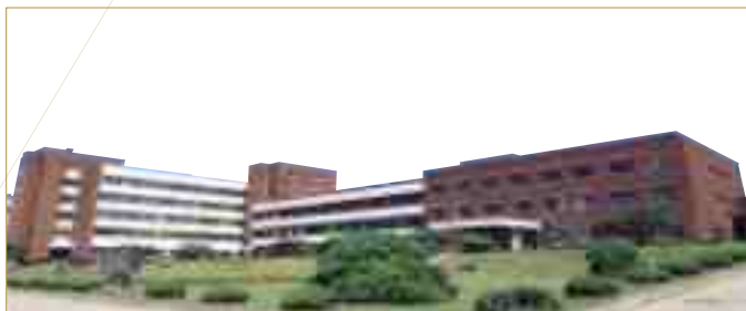
SK Chemicals R & D Center
