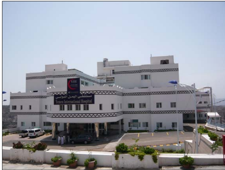
150 Bed Tertiary Care Hospital, Yemen
